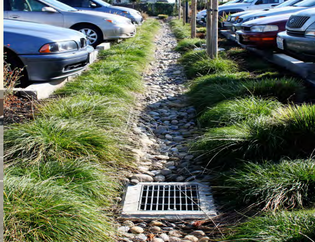
Bioswales, rain gardens, and native landscaping provide site-level stormwater benefits
